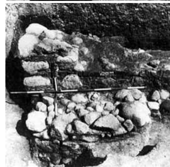
Fundamenty domu Kochanowskich The foundation of the Kochanowski family's house (fot. / photo: archiwum Stowarzyszenia / from the archives of the Association)
